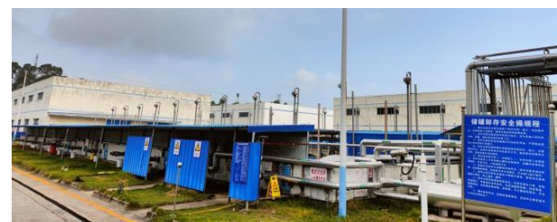
Underground Storage Tank
