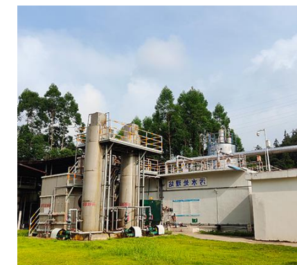
Sewage treatment station
